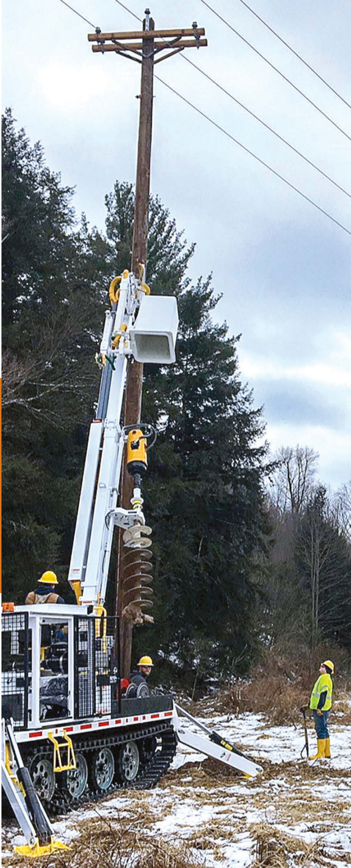
OFF-ROAD EQUIPPED. Claverack's Tunkhannock line crew uses the co-op's new UTV track digger derrick to replace a pole in the Springville area that had been washed out by flooding. The track machine, which is shared by all three Claverack districts, was put into service in February 2019. The track machine enables crews to access off-road locations with a digger and bucket.
