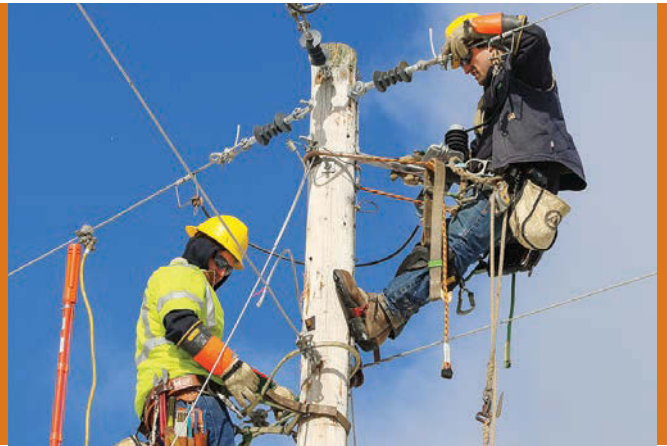
SYSTEM IMPROVEMENTS. Apprentice linemen David Gardner, left, and Kyle Urban team up to restructure the equipment on a pole as part of a line relocation project near Lawton in Bradford County.
